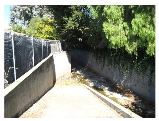
Figure 32: Permanente Creek at Villa Street Looking North Showing a Maintenance Access Ramp Leading Directly to the Creek
