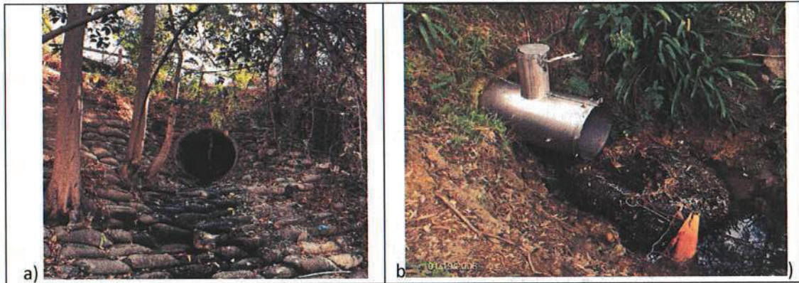
Figure 3. Trash monitoring outfall (a) and NetTech device (b) to be installed at outfall.
