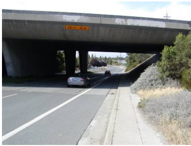
Foothill Boulevard under crossing of I-280
