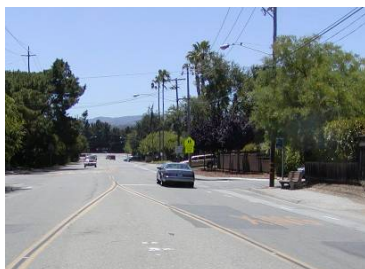
Existing conditions on Grant Road looking northbound
