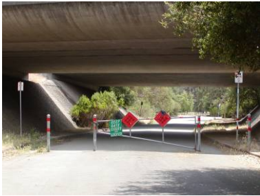
Connection from St. Joseph Avenue, under I-280, to Rancho San Antonio Park
