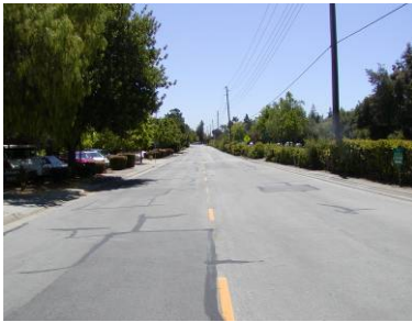
Existing conditions on Grant Road adjacent to Foothill Expressway
