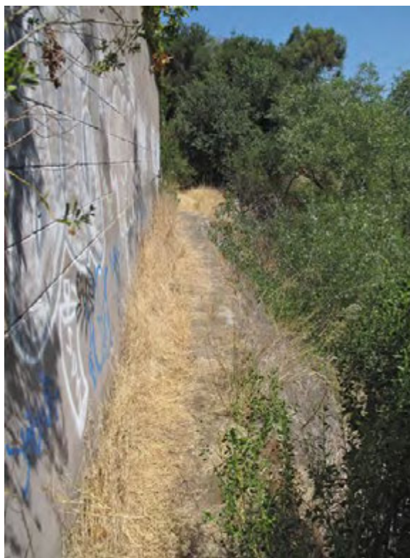
Inadequate top-of-bank behind the soundwall along State Route 85 at a channel meander.
