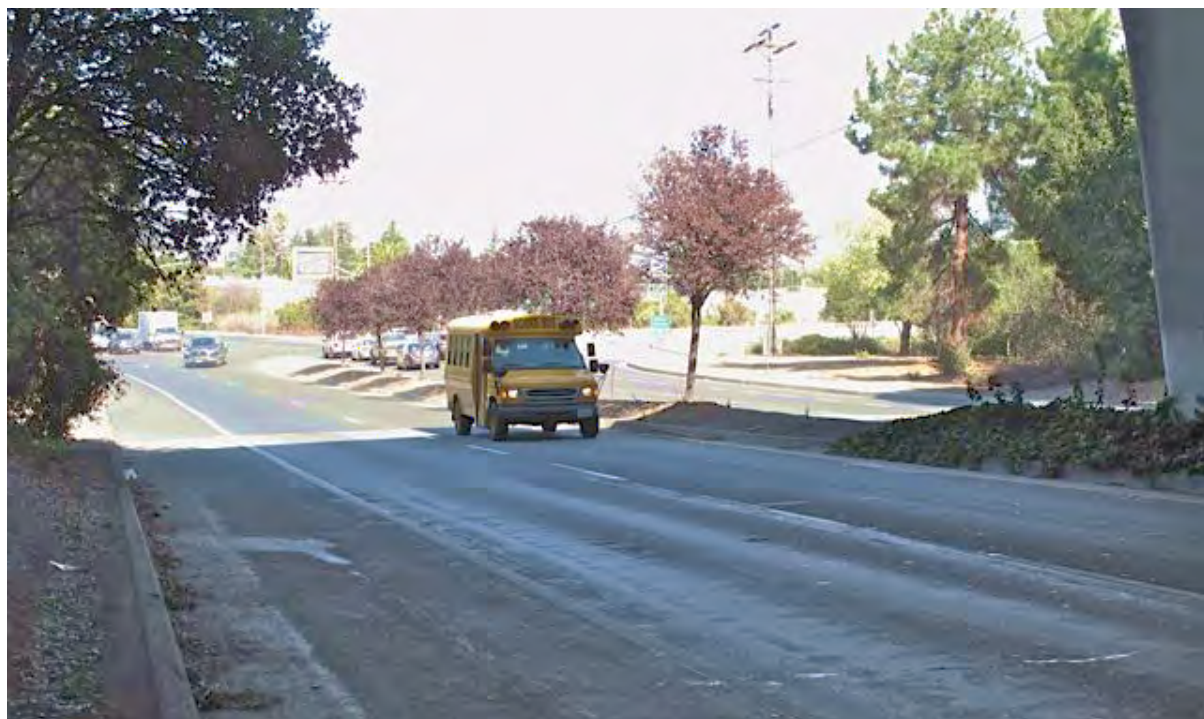
Foothill Expressway beneath Interstate 280.
