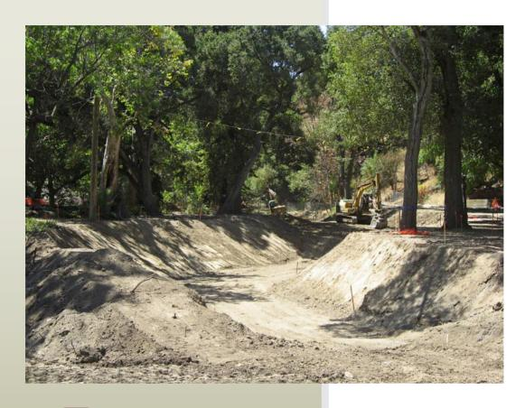
The creek channel was excavated, with an alignment tailored to the locations of trees. The entire team worked long hours during this time and the work progressed well
