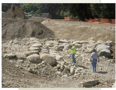
The new banks were also constructed in some areas with logs and rootballs placed in a manner to stabilize the slopes and channel. The channel restoration plan used logs and boulders as major engineered elements
