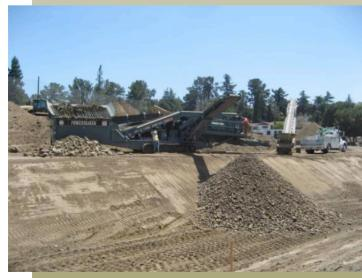
from the site. In all, over 6,000 cubic yards of existing material was reused on site in the channel restoration process.
