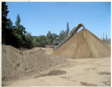
Fill with particular qualities, known as "engineered fill", was needed to create the new channel and banks. The project designers estimated that more than 1,000 cubic yards of import might be needed to amend the onsite soil to make it suitable for this purpose. Ferma Corporation used specialized equipment during the earthwork process. The equipment sorted, screened and proc-
