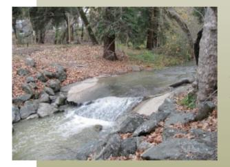
A fter fish relocation and dewatering, another important task was removal of the low-flow crossings in the channel. Riprap was salvaged and reused
