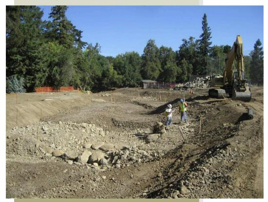
The new channel through the former parking lot took shape, and the bed was filled with graded gravel and cobble
