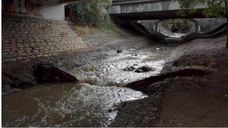
The fish passage project improves conditions for fish migrating upstream.
