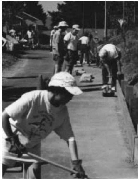
The Synopsys Green Team at work taming an embankment.
